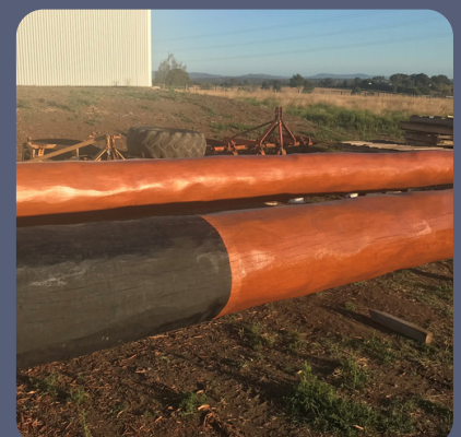
4 Bitumen paint application and softfall marker
